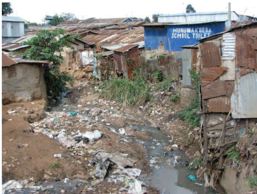
Plate 3: Note the School Pit Latrine and Shanties elected on the River Bank
